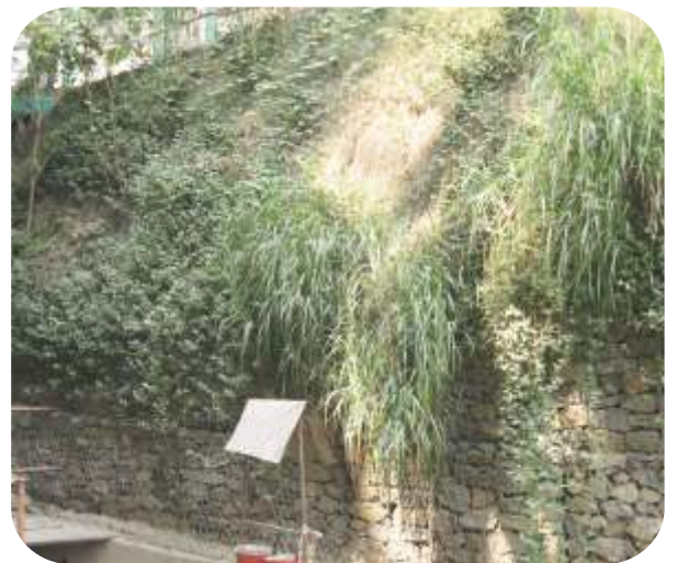
GREEN TERRAMESH SYSTEM FOR STEEP SLOPE STABILIZATION
