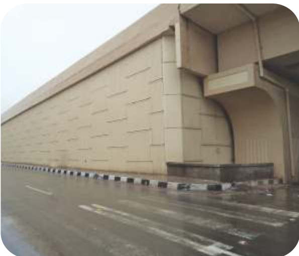
PARAWEB REINFORCED SOIL WALL
