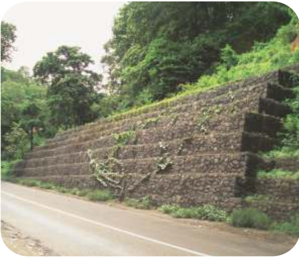
GABION RETAINING WALL
