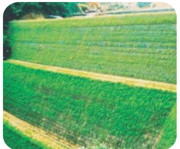
PARAGRID REINFORCED SLOPE
