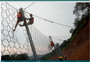
Figure-4 Installation of Primary Interception mesh (MacRing)
