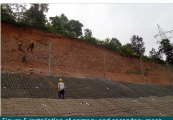
Figure-5 Installation of primary and secondary mesh (MacRing + DT mesh)
