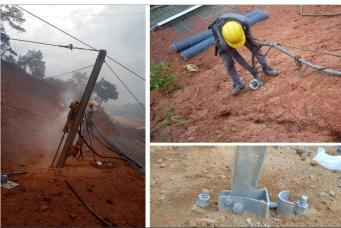
Figure-2 Activities related to installation of barrier posts
