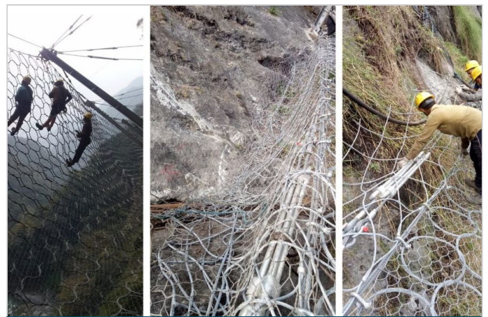
Figure-4 Installation of interception meshes and skirting arrangement
