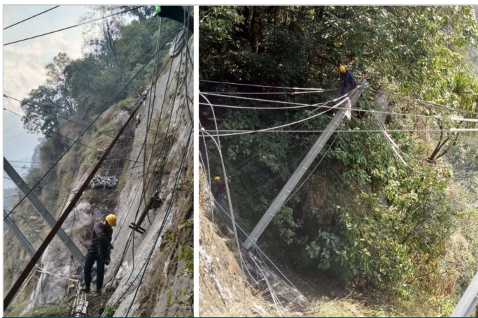
Figure-3 Installation of posts
