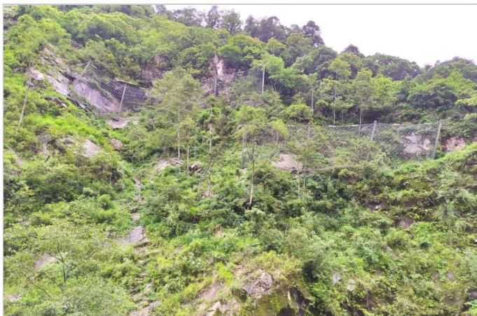
Figure-5 Installed rockfall barriers above ST-1 portal
