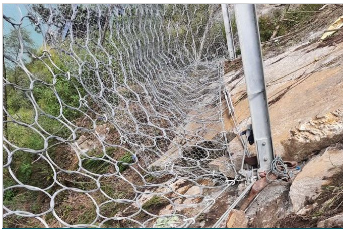
Figure-3 Installation of interception meshes (primary and secondary) in progress
