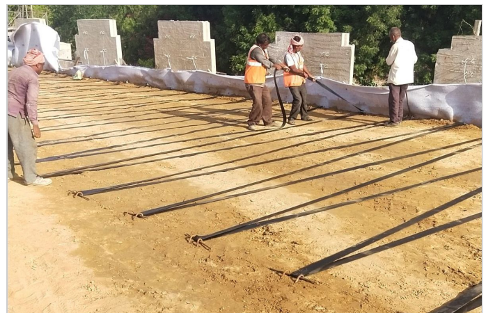
PARAWEB LAYING IS IN PROGRESS
