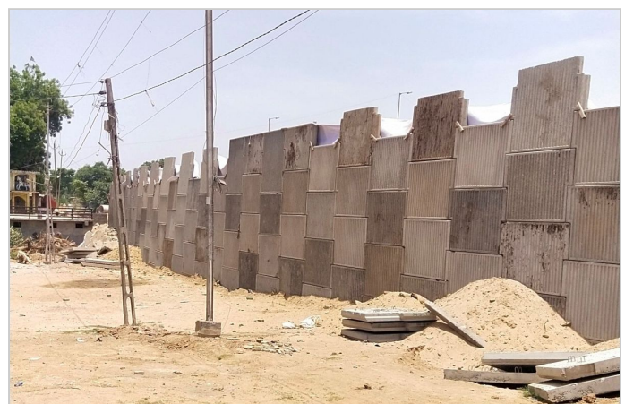
ERECTION OF LOWER TIERED WALL IN PROGRESS
