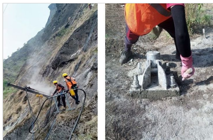
Figure-1 Activities related to installation of barrier posts
