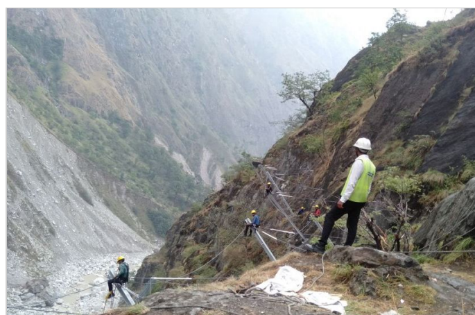
Figure-2 Rockfall barrier post erection completed
