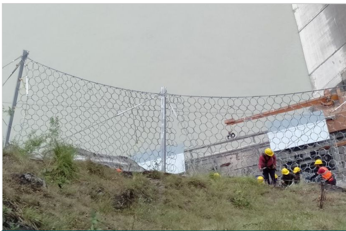
Figure-3 Installation of primary interception mesh (MacRing)
