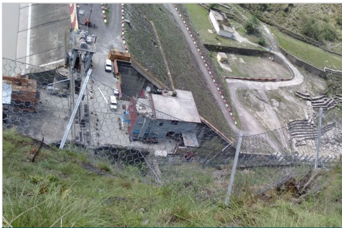
Figure-5 Top view of installed Rockfall barrier
