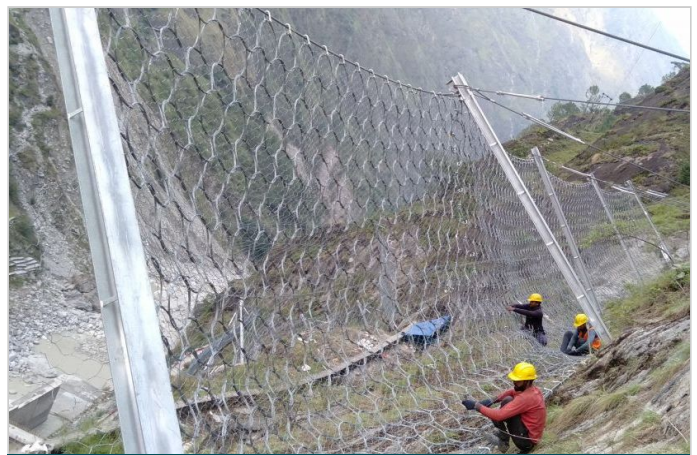
Figure-4 Installation of Secondary mesh (DT mesh) on upslope side of MacRing
