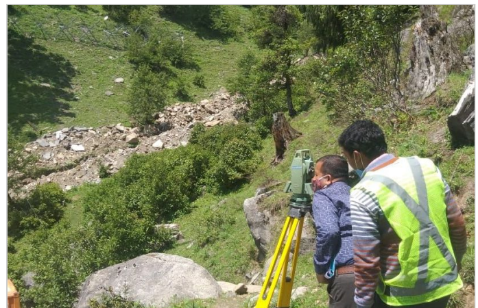
Figure-1 Survey ongoing for alignment verification
