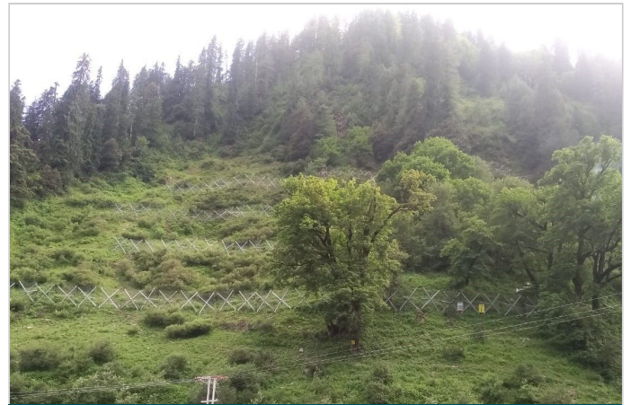
Figure-6 Multiple lines of Snow ErdoX units installed
