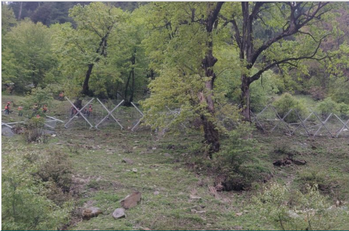
Figure-3 Placement of Snow ErdoX units along stipulated alignment
