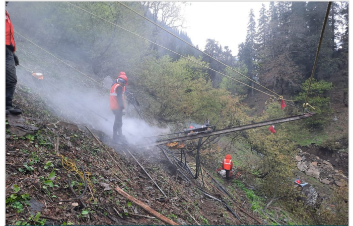
Figure-4 Drilling for nails (foundation) in progress
