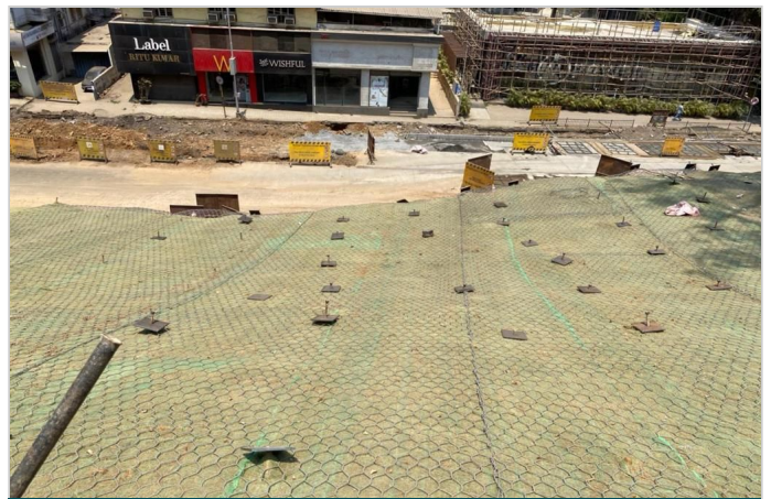
Figure-6 Meshes including DT Mesh installed over slope
