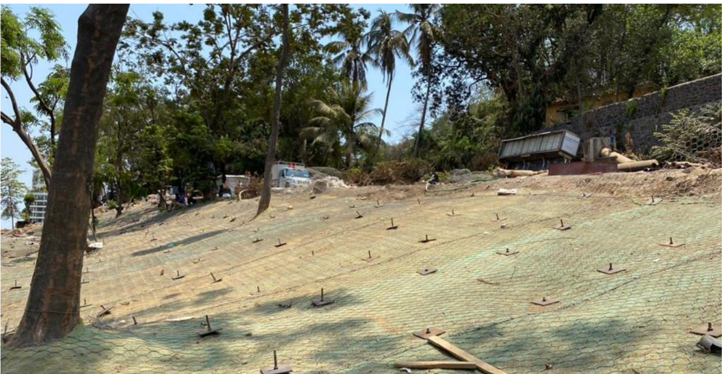
Slope after installation of meshes
