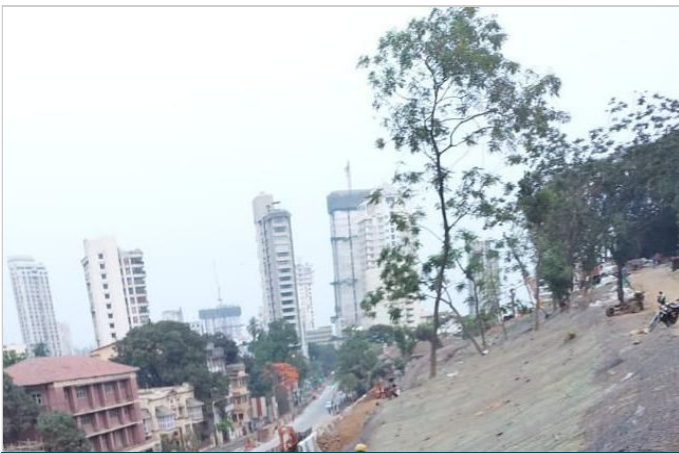
Figure-5 Meshes including DT Mesh installed over slope
