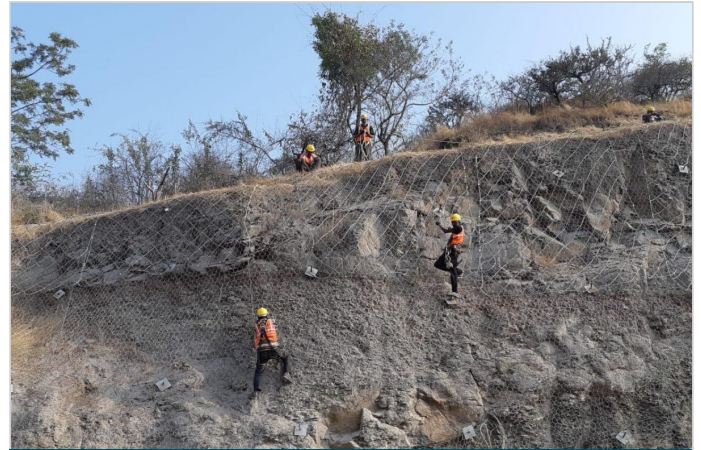
Figure-4 Installation of HEA Panel (over DT Mesh) in progress
