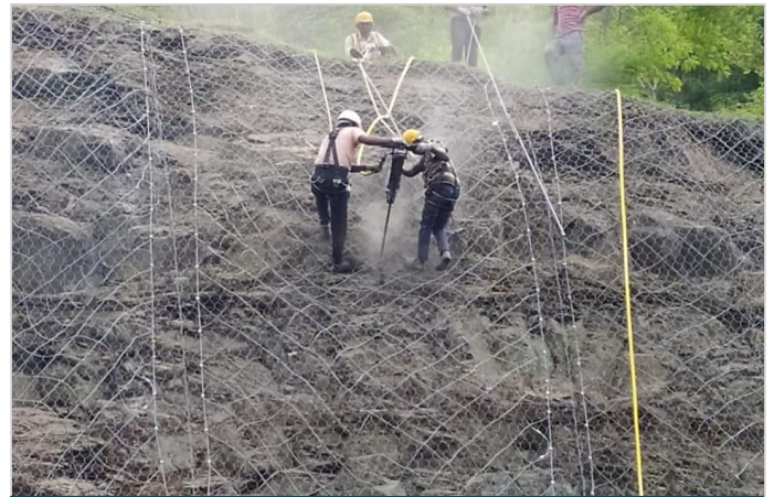
Figure-6 Installation of surface nails in progress
