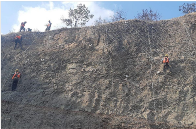
Figure-5 Installation of HEA Panel in progress
