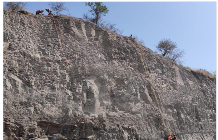
Figure-1 Installation of DT mesh as secondary mesh in progress
