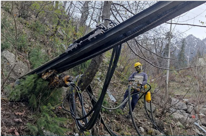
Figure-3: Drilling operation for anchors
