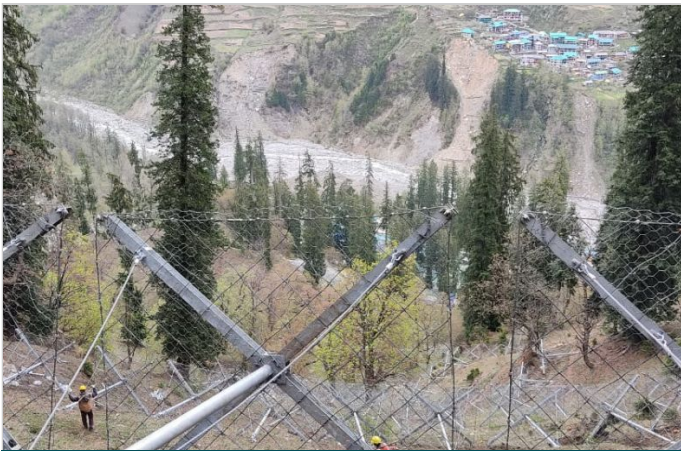
Figure-5: Multiple lines of Snow ErdoX installed
