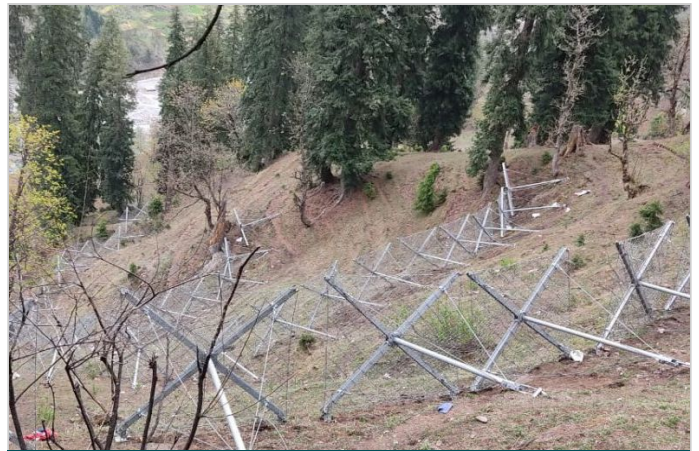
Figure-6: Multiple lines of Snow ErdoX installed
