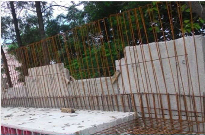
CONSTRUCTION OF RCC WALL & ITS CONNECTION WITH PRECAST FASCIA PANEL
