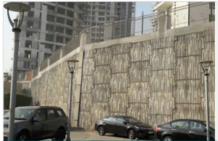
COMPLETE VIEW OF RS WALL & BUILDINGS CONSTRUCTED OVER FORMATION LEVEL
