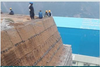
Photo 5: Installation of Green Terramesh units
