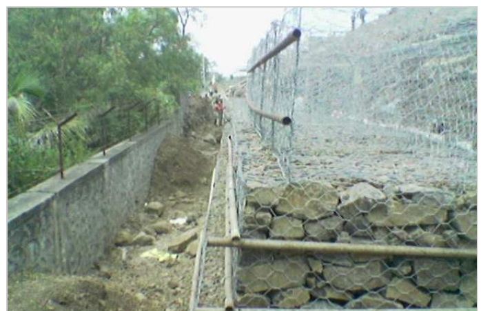
Photo 2: Maintaining horizontal and vertical alignment of wall using rods
