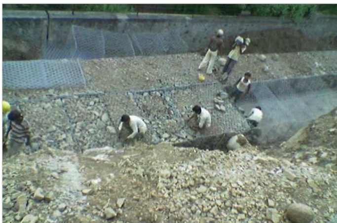
Photo 3: Filling of gabion boxes
