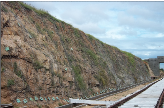
HEA Panel Installation Completed
