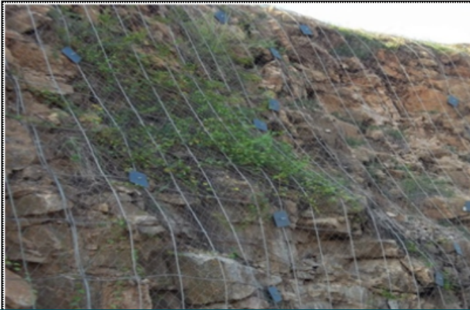
HEA Panel Installation Completed
