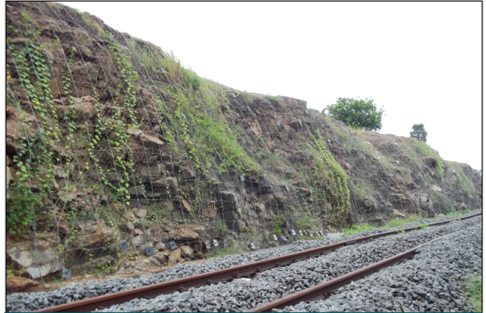
HEA Panel Installation Completed
