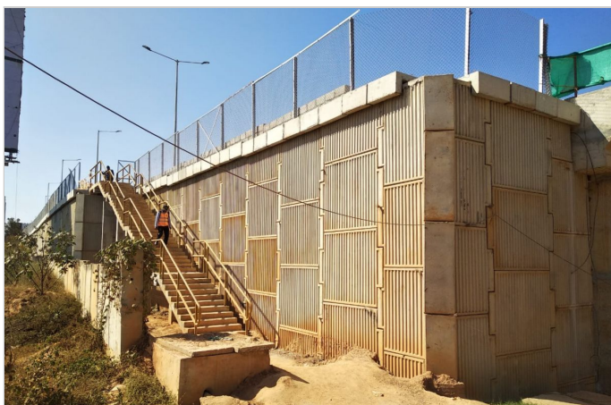
Photo 5: After completion of RS wall and fencing over it
