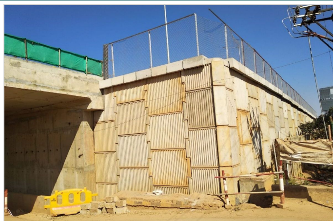
Photo 4: Merging Portion of newly constructed RS wall with existing structure
