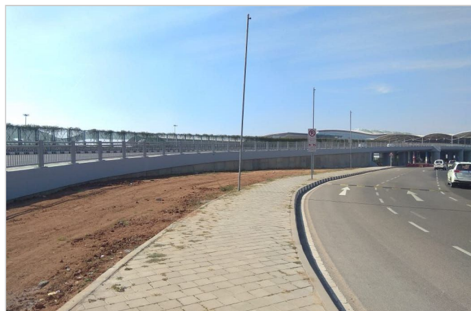
Photo 6: Completed RS wall structure
