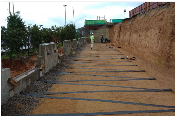
Photo 3: Connecting Paraweb to cavity-connector & fixing with J-hooks on rear end
