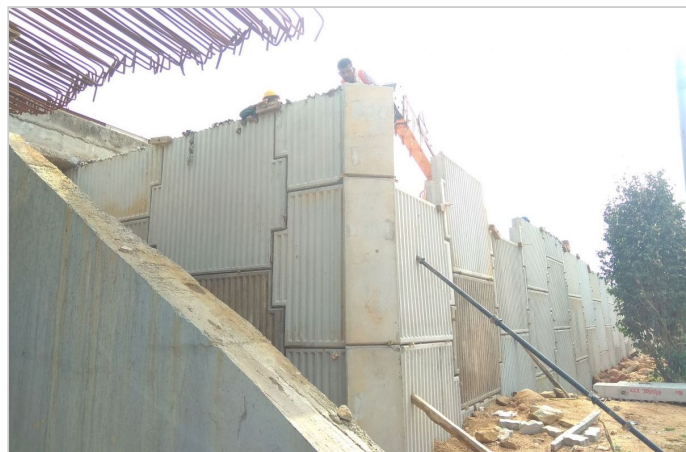
Photo 4: Corner facia panels joining longitudinal wall & cross wall
