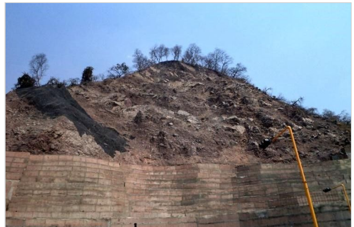
Photo 1: Photograph showing variable strata present at site
