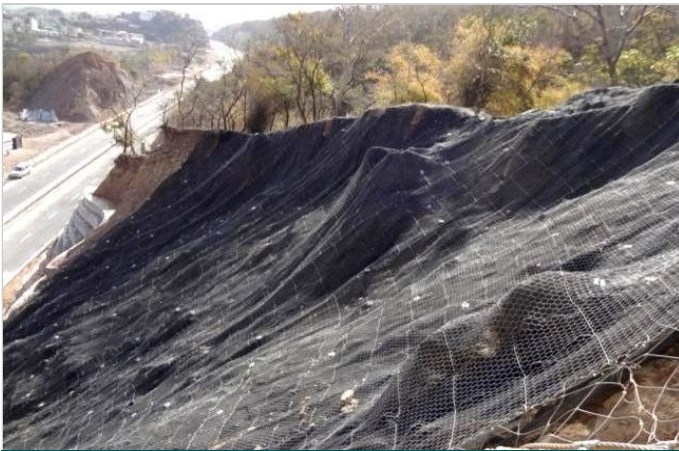
Photo 5: Photograph showing MacMat R used in conjunction with Steelgrid BO
