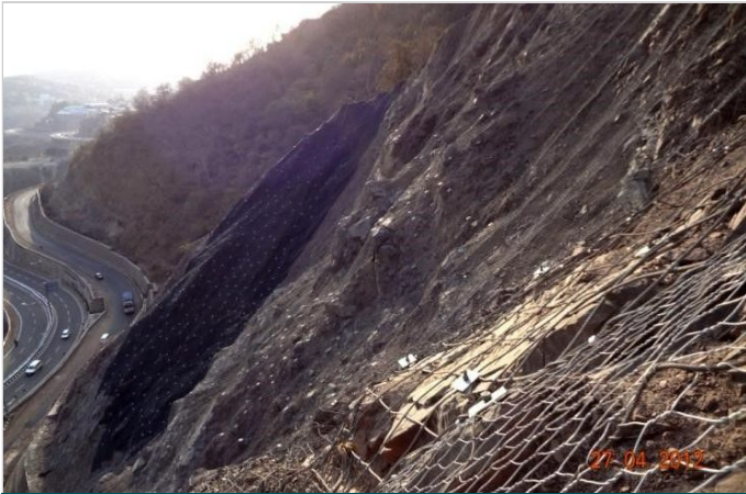
Photo 3: Photograph showing Steelgrid BO on rocky slope - April 2012
