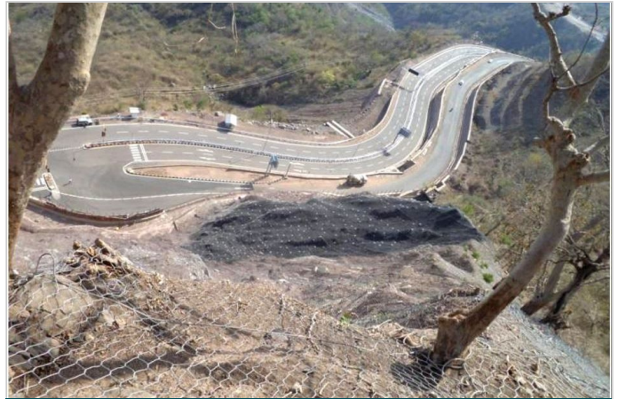
Photo 4: Photograph showing Steelgrid BO on slope
