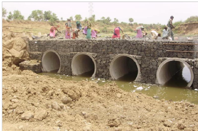
Photo 6: Construction of gabion wall
