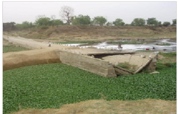
Photo 1: Site Before Construction- RCC Structure failure
