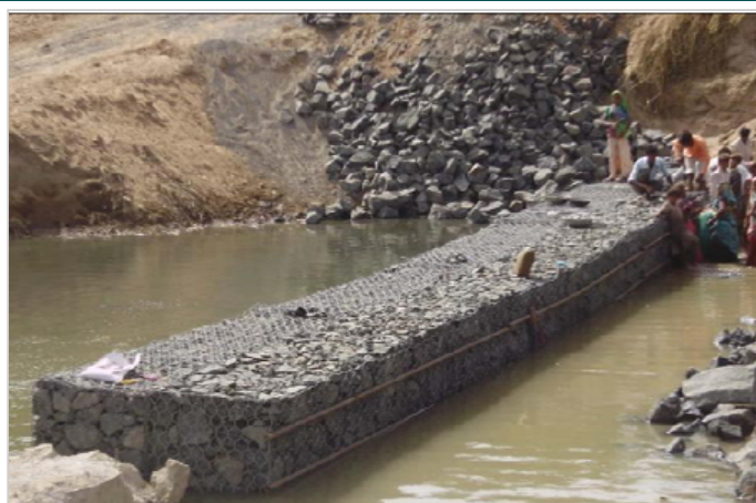
Photo 4: Gabion layers placed in position
