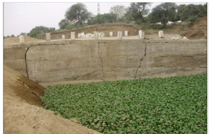
Photo 2: Site Before Construction- RCC Structure failure
