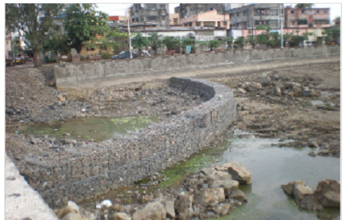
Photo 1: Construction of gabion wall, Digha lake
