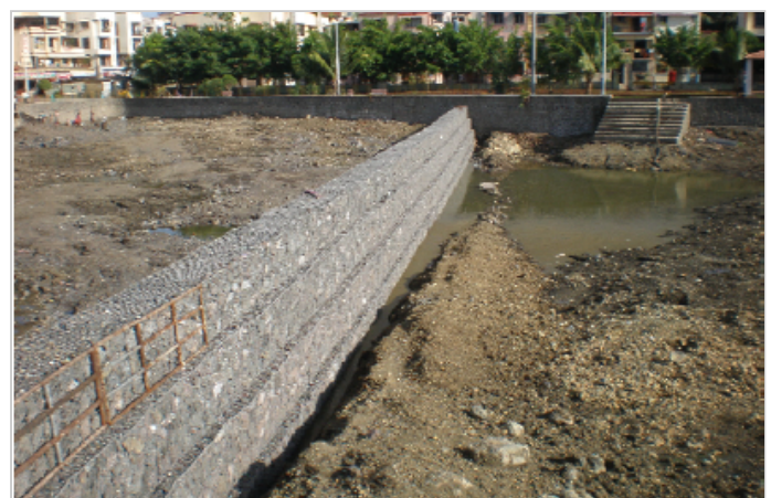
Photo 2: Partition gabion wall, Nerul lake
