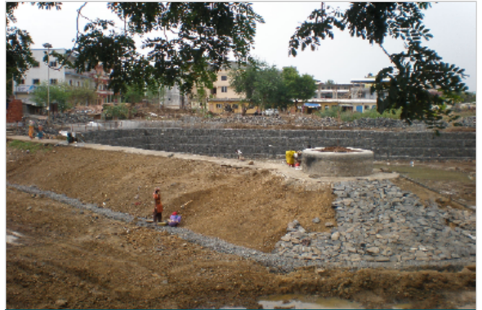
Photo 4: Gabion wall, Gunali lake
