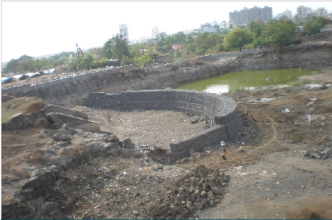
Photo 3: Partition gabion wall, Ghansoli lake
