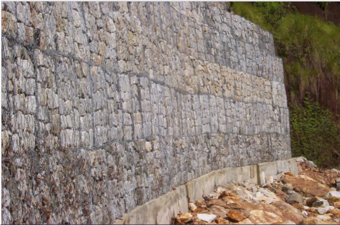
Photo 3: Placement of stones in hexagonal wire crates
