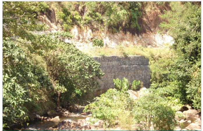
Photo 6: Gabion wall after 2 years
