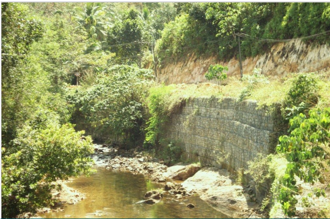
Photo 5: Gabion wall after 2 years
