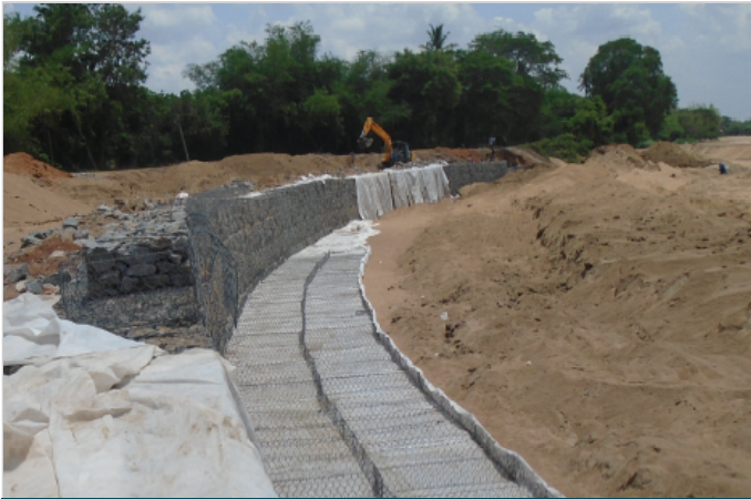
Photo 3: Construction of launching apron using mattress
