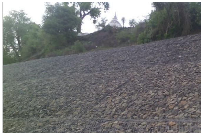
Photo 4: Bank slope after execution of mattress
