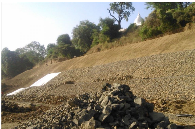
Photo 3: Laying mattress over the slope
