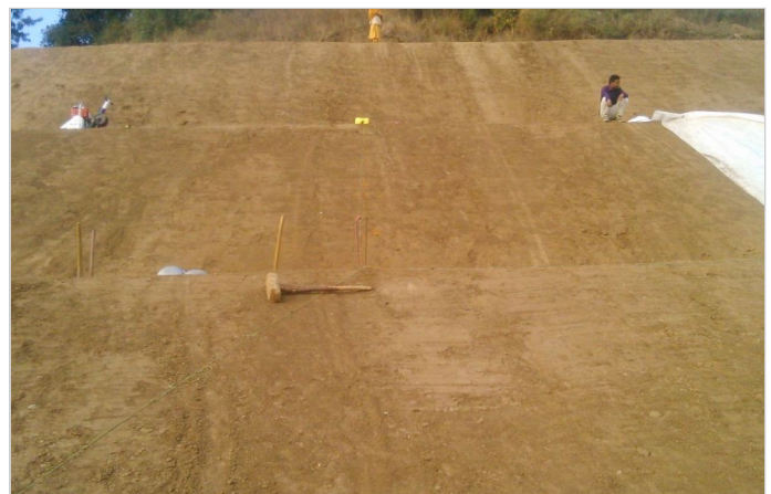
Photo 2: Preparing slope with proper surface compaction
