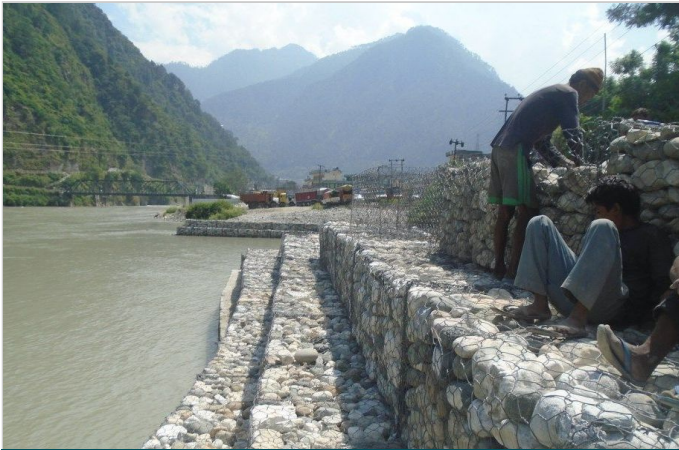
Photo 3: Afflux bund during construction
