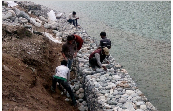
Photo 4: Gabion filling during construction
