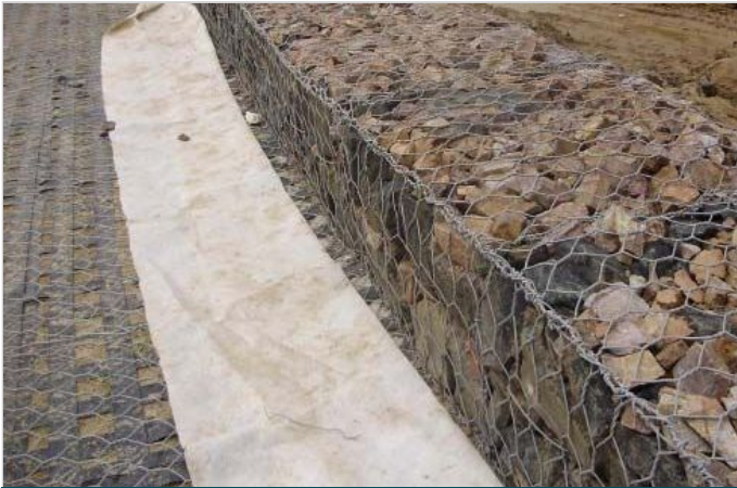
Photo 3: During construction- Laying of geotextile-Terramesh system
