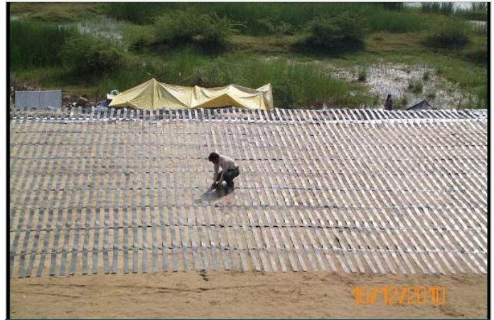
Photo 4: During construction- Laying of ParaLink-Terramesh system
