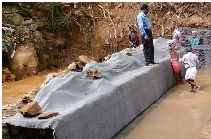
Photo 2: MacLine GCL placed in between gabions
