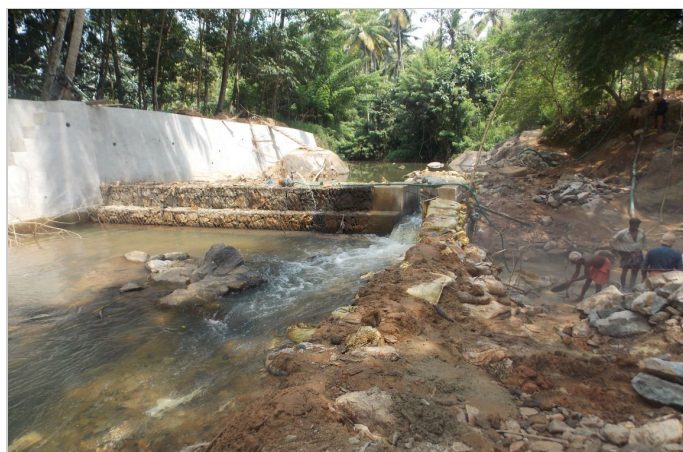
Photo 1: Construction of check dam using Gabions and GCL
