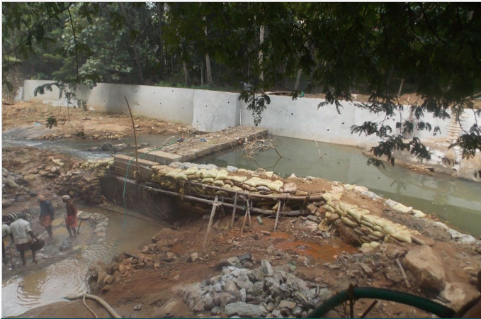
Photo 3: During construction of check dam
