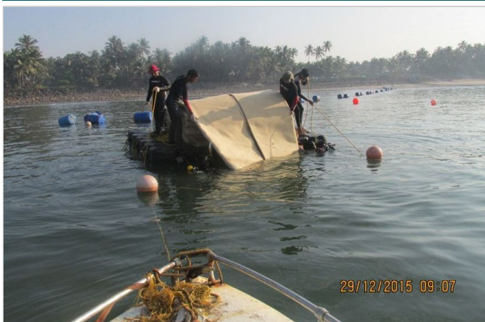
Photo 3: Placing of geotextile tubes
