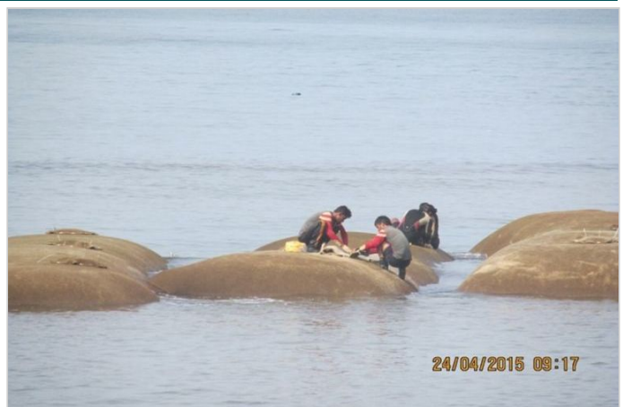
Photo 4: Closing of filler ports
