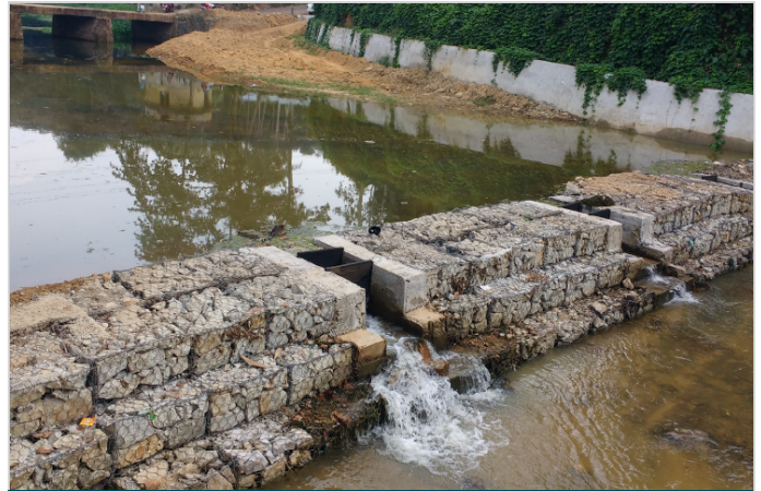
Photo 4: Completed structure with infiltration gallery on the upstream side
