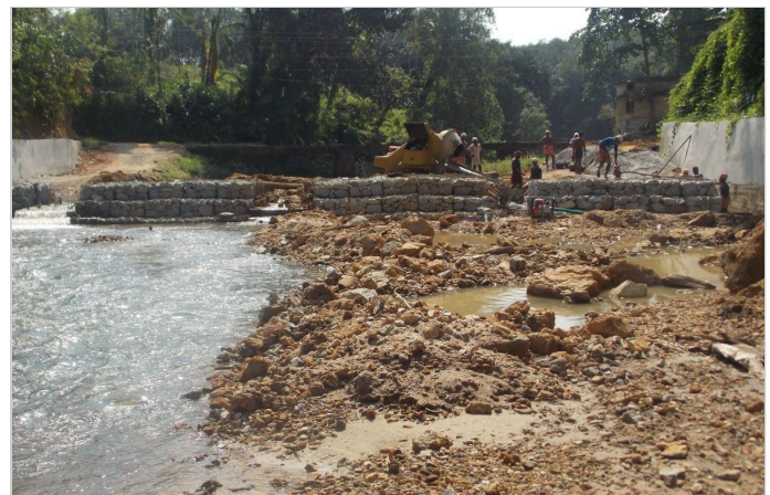
Photo 1: Construction of check dam using gabions and MacLine GCL
