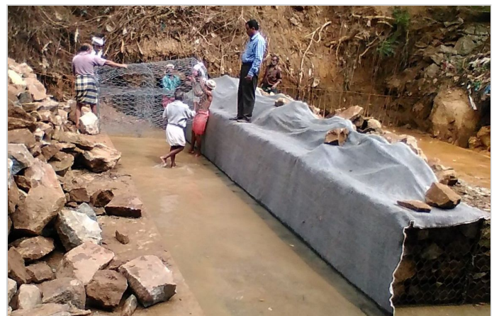
Photo 2: Macline GCL placed in between gabions
