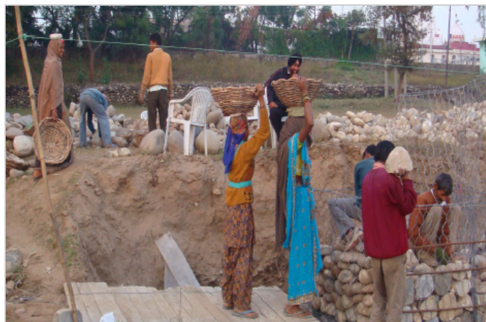
Photo 4: During construction- filling of gabions
