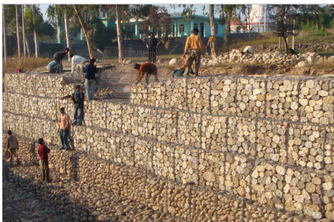
Photo 5: Wall near to completion- gabion mattress laid for scour protection
