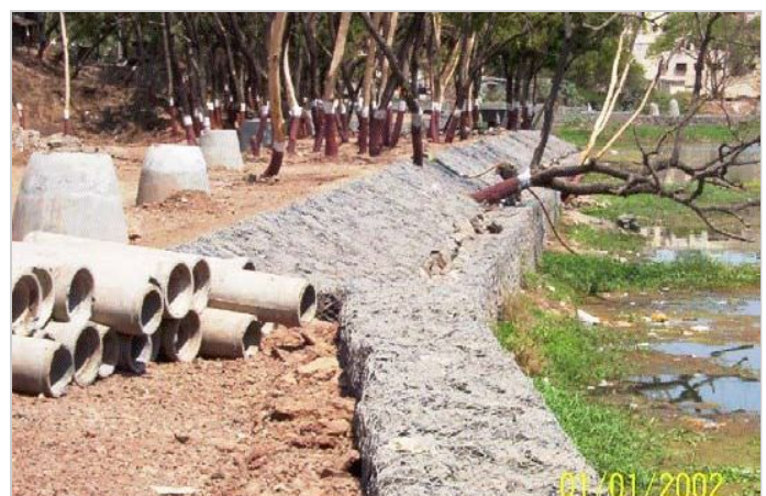
Photo 2: Reno Mattress for protection of top slope
