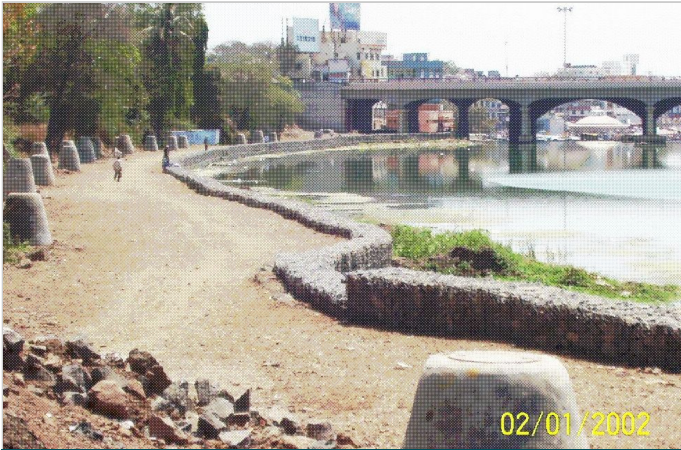
Photo 3: Lining of river bank with gabion retaining wall
