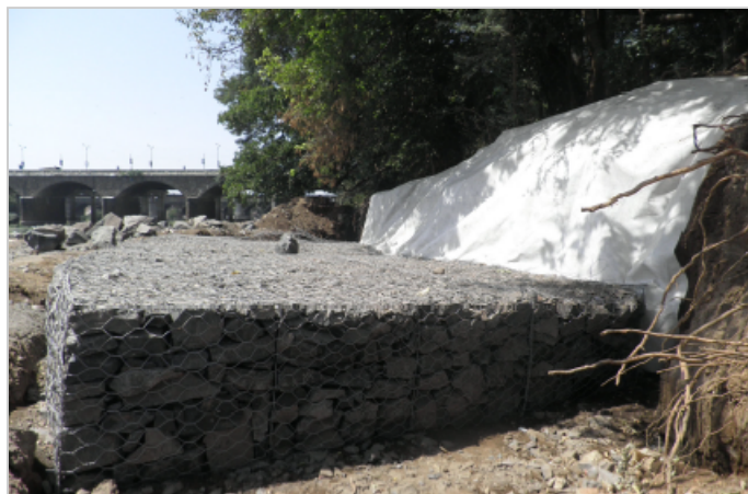
Photo 2: Construction of bottom layer
