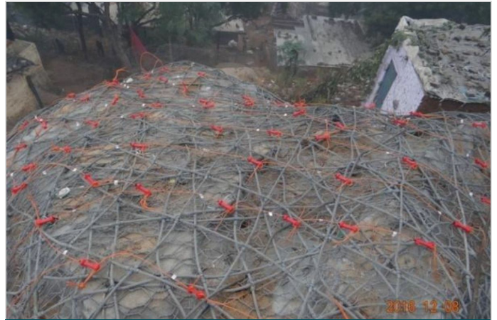
Figure 4- Catridge explosives and nonel units fixed above the boulder
