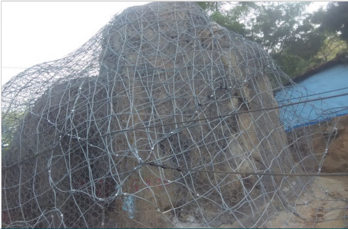
Figure 3- Boulder covered with the meshes and wire ropes anchored with nails
