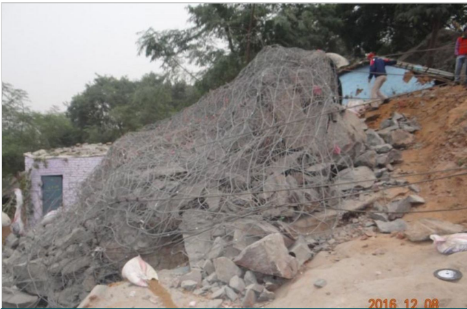
Figure 5- Boulder after blasting with mesh containing demolished fragments
