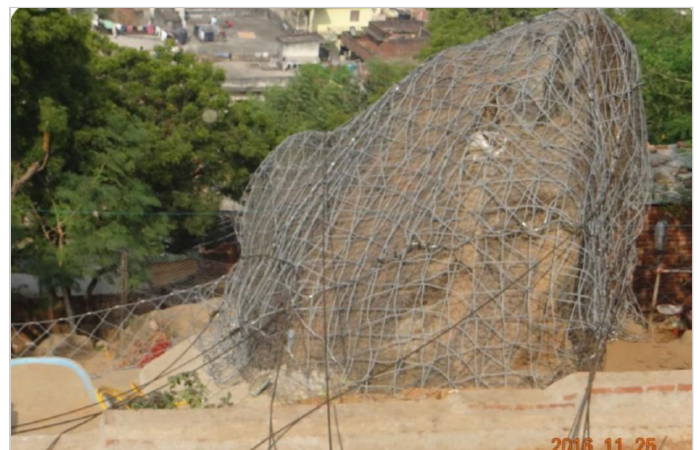
Figure 2- Boulder covered with the meshes and mesh fence on side
