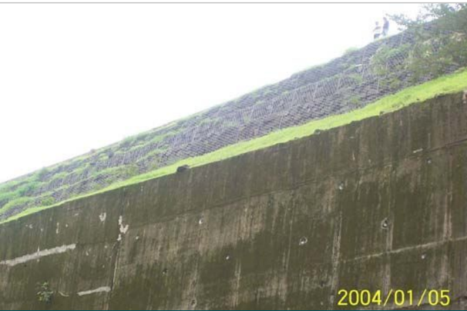
Photo 5: Gabions on the valley side where global stability was critical
