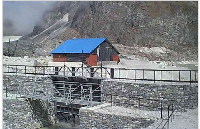
Photo 4: Undersluice gate built with gabions
