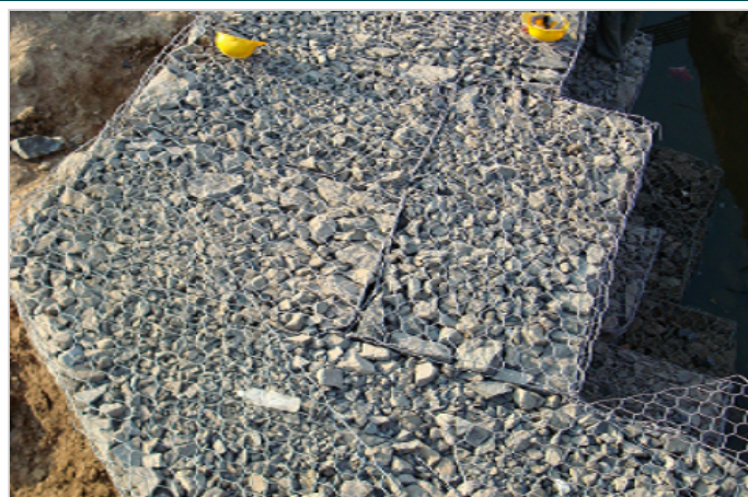
Photo 4: During Construction - Gabion Layer, Placed in Skew
