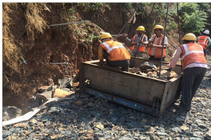
Figure 4-Placement of boulders for fill
