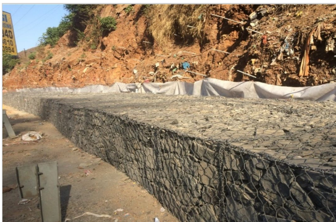
Figure 3-Bottom Gabion row completed (non-woven geotextile visible behind)
