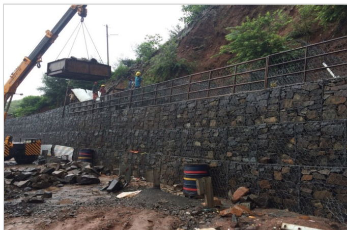
Figure 6-Soil Nailing with gabion facia
