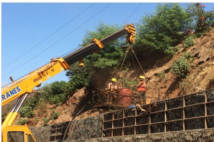
Figure 5-Nail installation of intermediate nail rows
