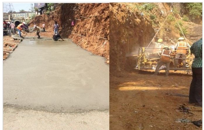
Figure 2-PCC base preparation(left), Drilling of bottom nail (right)
