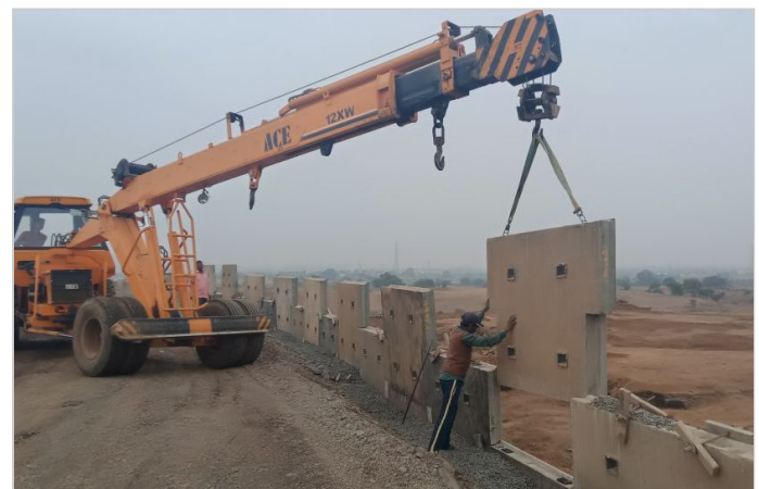
Photo 1: T-shaped panels being erected with the help of Hydra
