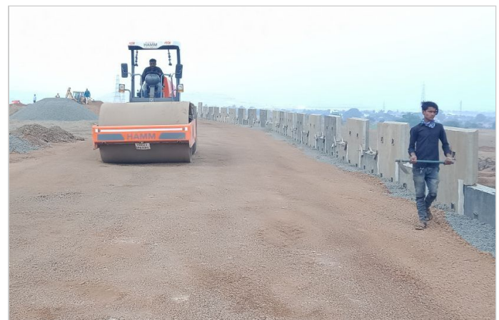
Photo 2: Bed being prepared for ParaWeb reinforcement laying
