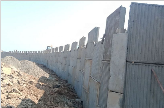
Photo 3: RS wall constructed in a curve
