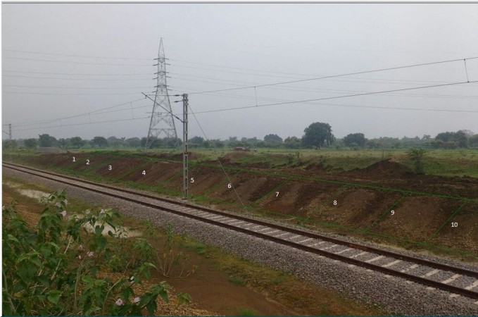
Photo 3: Division of slope into multiple bays
