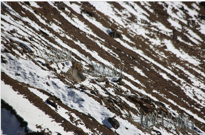
Figure 5. Installed Erdox units (during snowfall)
