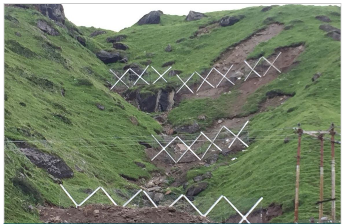
Figure 4. Installed Erdox units
