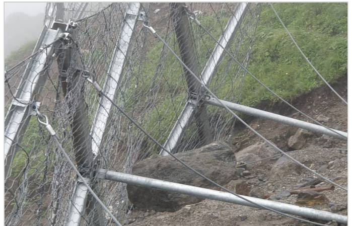
Figure 6. Debris trapped by Erdox immediately after installation
