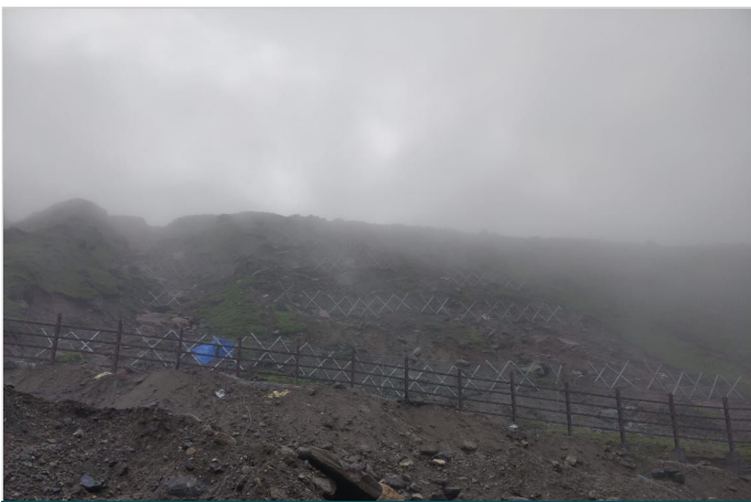
Figure 3. Installed Erdox units & protection fence
