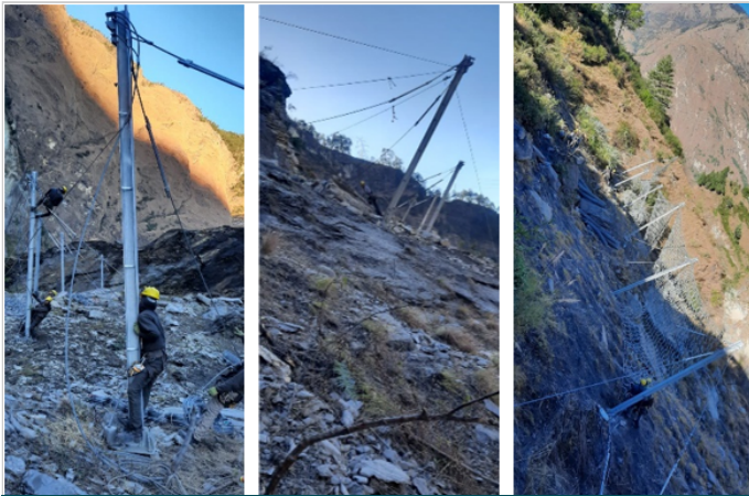
Figure-3. Installation of Rockfall barrier
