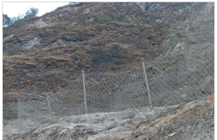
Figure-6. View of installed Rockfall barrier
