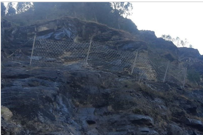
Figure-5. View of installed Rockfall barrier
