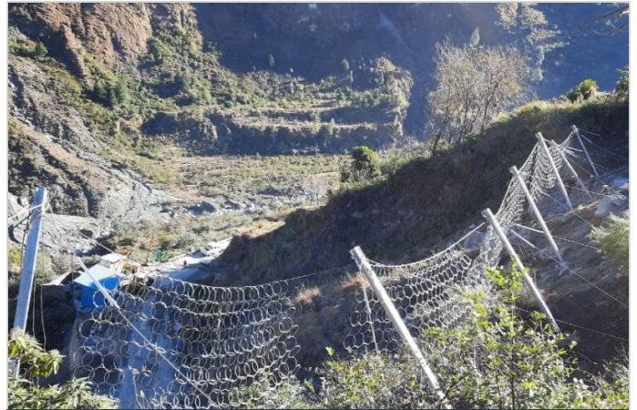
Figure-4. Erection of Rockfall barrier
