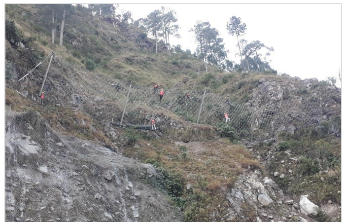
Figure-2. Installation of Rockfall barrier
