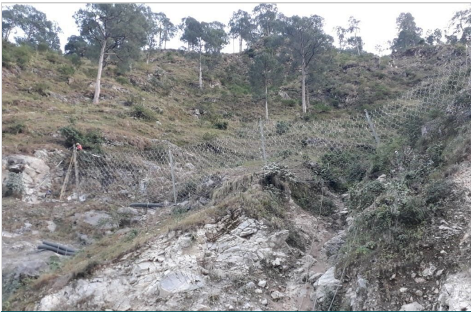
Figure-5. Front view of Rockfall barrier
