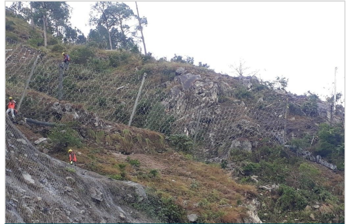
Figure-4.Installation of Rockfall barrier
