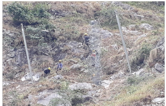
Figure-1. Installation of Rockfall barrier
