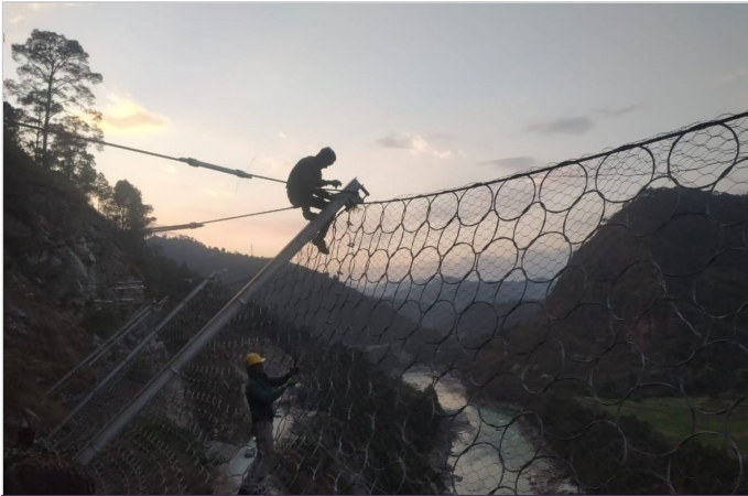
Figure-3.Installation of Rockfall barrier
