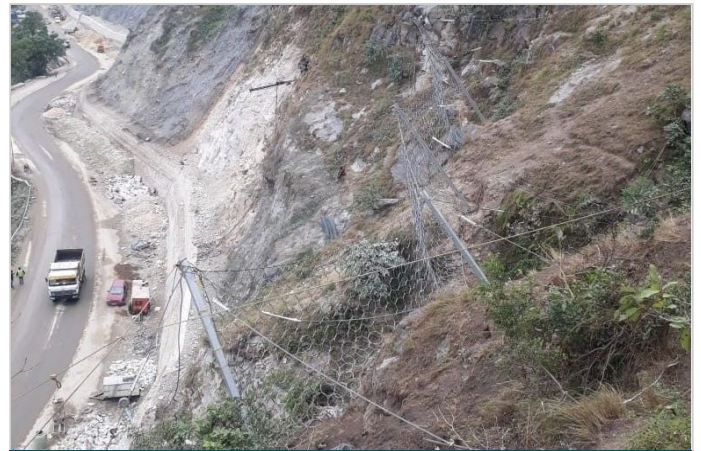
Figure-6. Top view of Rockfall barrier
