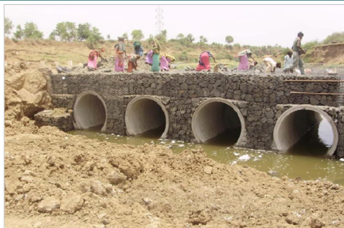
Photo 4. Construction of Gabion wall
