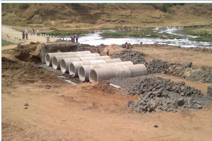
Photo 3. Pipes placed in position
