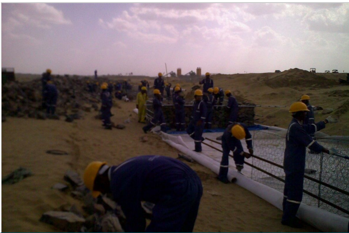
Photo 3: Alignment for placing Gabion boxes using bamboo
