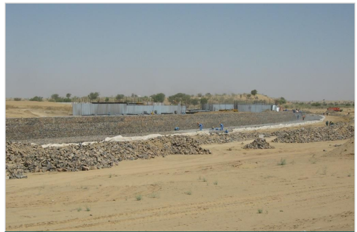
Photo 6: After construction Gabion & launching apron
