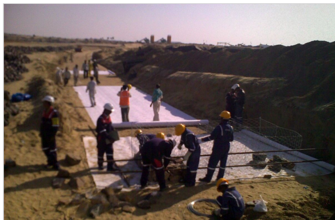
Photo 2: Placing of Gabion boxes over geotextile
