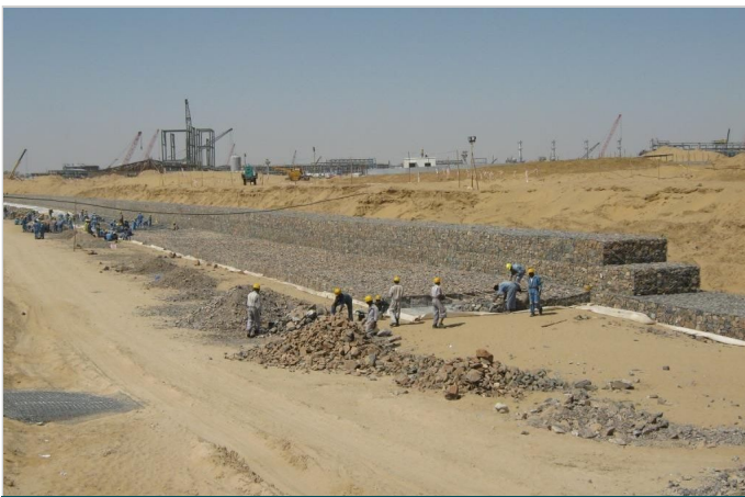
Photo 5: Gabion wall & laying of launching apron of 0.5 m thick
