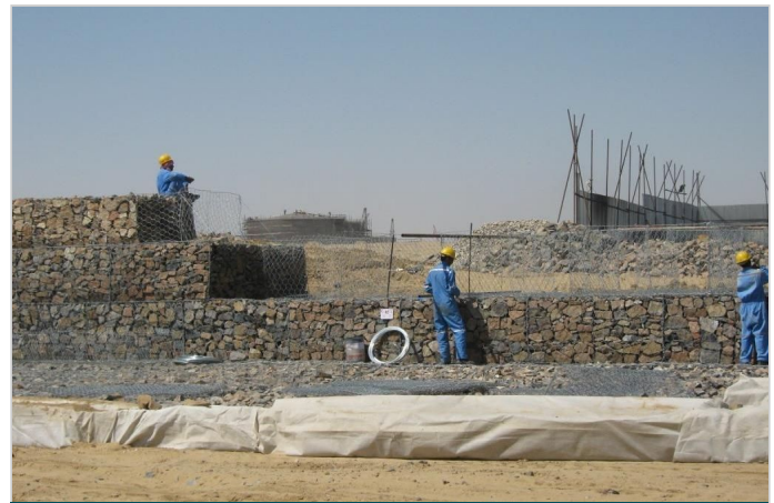
Photo 4: Gabion boxes placed in different layers
