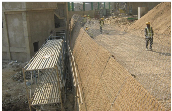
Photo 4: During construction of Green Terramesh® system
