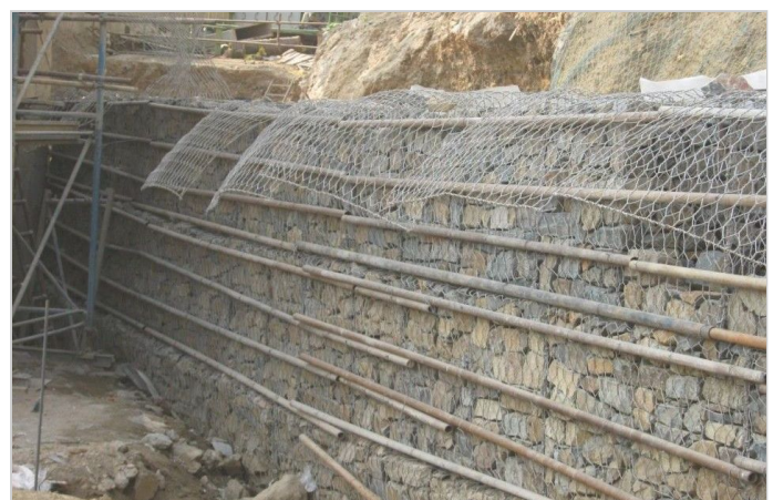
Photo 2: During construction of Terramesh® system
