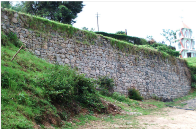
Photo 5: Vegetated Gabion walls after completion of one year
