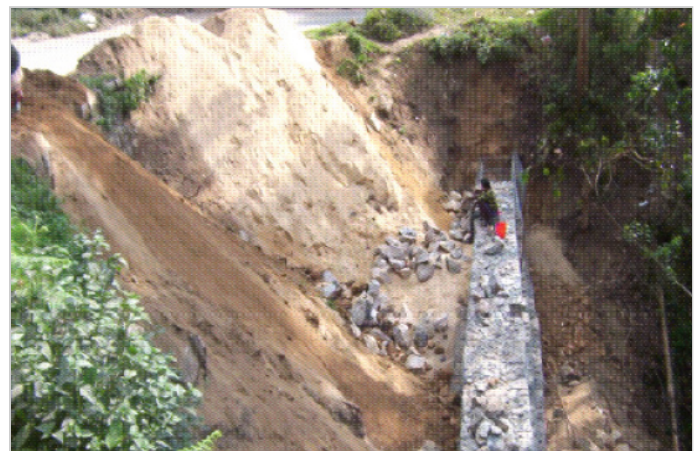
Photo 2: Gabion wall construction
