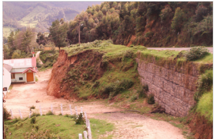
Photo 6: Vegetated Gabion walls after completion of one year
