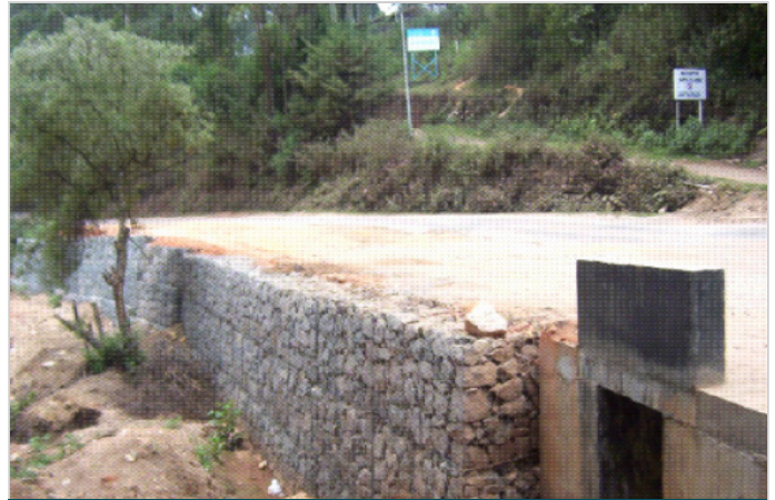
Photo 4: Culvert protection under construction stage
