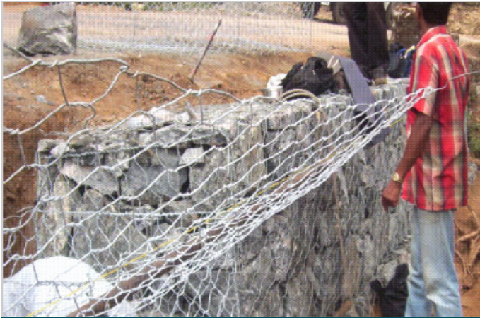
Photo 3: Gabion filling during construction
