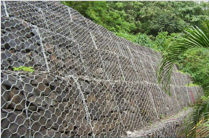
Photo 3 : Construction of Gabion wall behind club house
