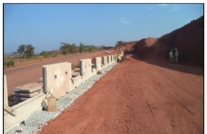
Photo 2: Compacted layer with cavity connector connections embedded in panels
