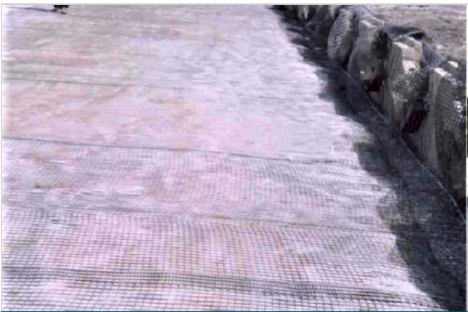
Placing of panels and Geogrid
