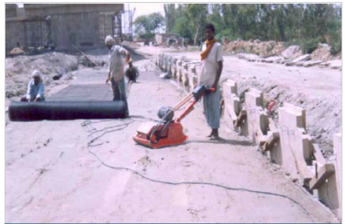
Photo 4 : Placing of Structural fill and compaction
