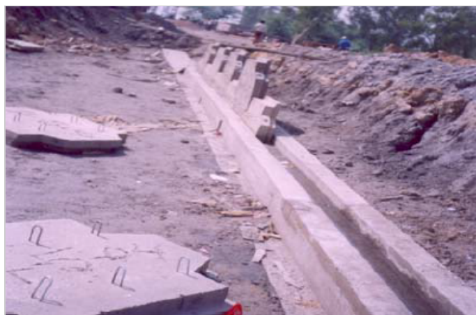
Photo 1: Construction of leveling pad
