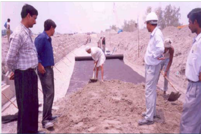
Photo 3 : Laying of Geotextile
