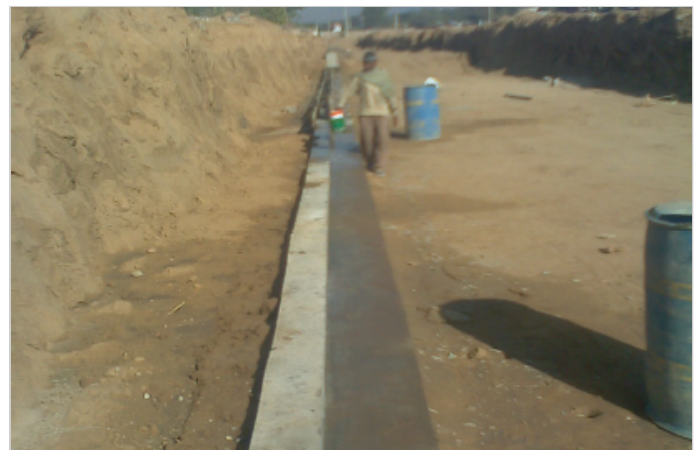
Photo 1: Construction of leveling pad
