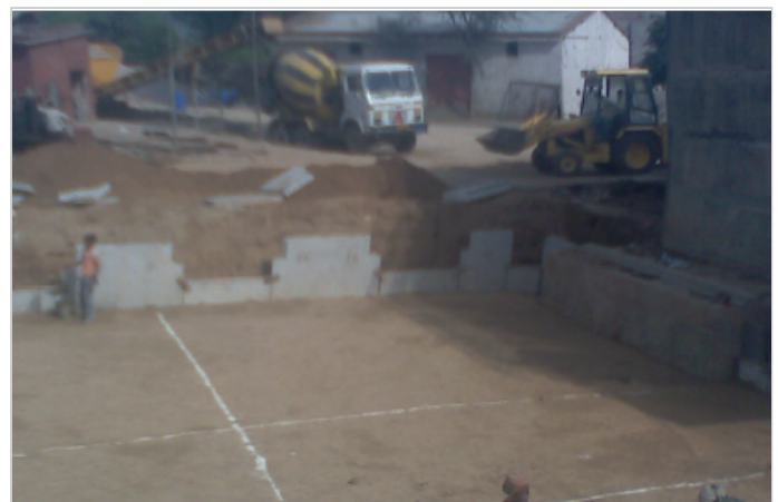
Photo 2: Erection of fascia panels
