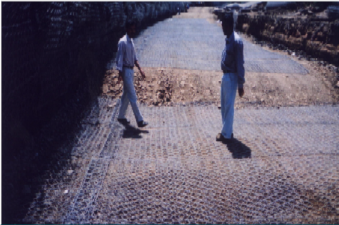
Photo 3: Laying of DT mesh
