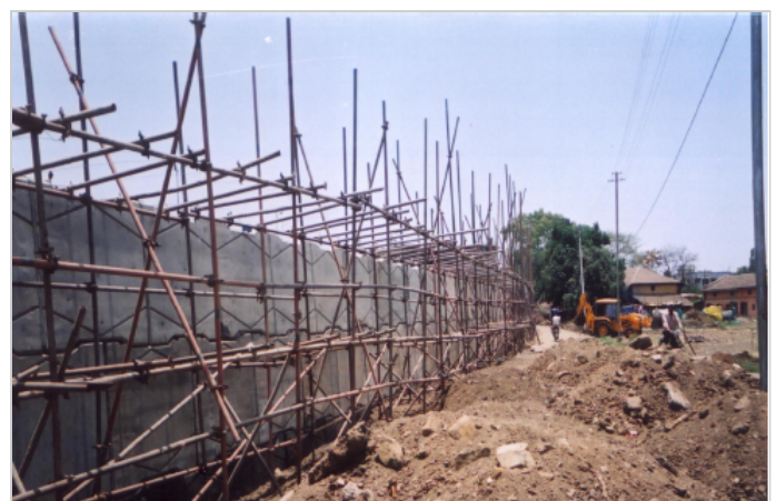
Photo 2 : Erection of fascia panels
