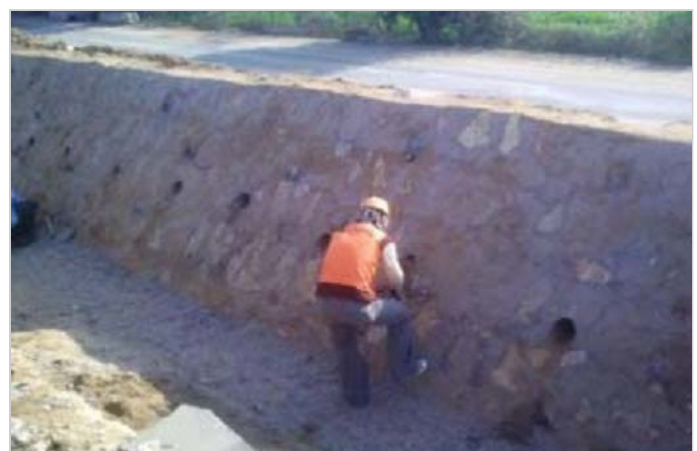
Photo 2: Dressing of protrusions
