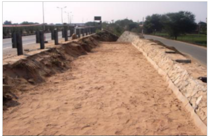
Photo 4: Placement of backfill till top of wall
