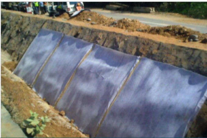
Photo 3: Placement and joining of MacDrain®
