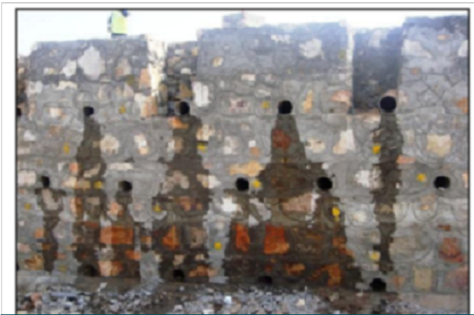
Photo 5: Seepage noted from weep holes
